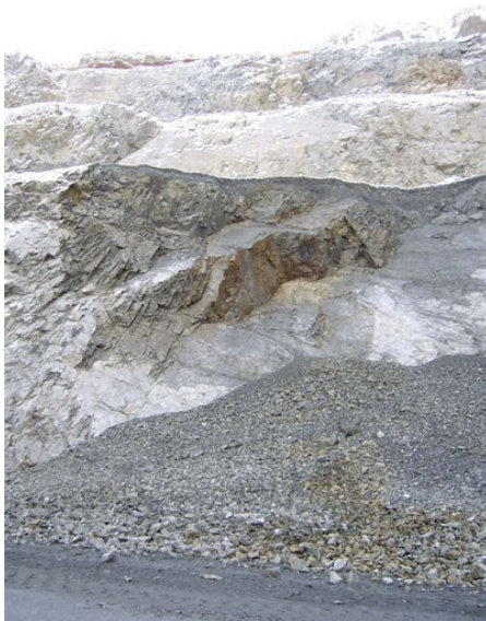
The slope after the failure
